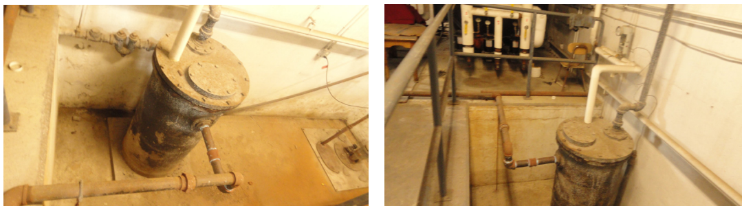
Photo 10: Existing tank receiving condensate
