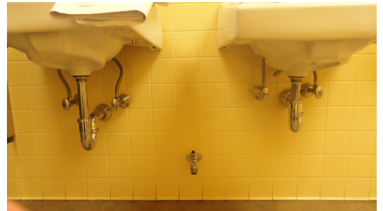
Non-ADA Lavatories and without pipe insulation
