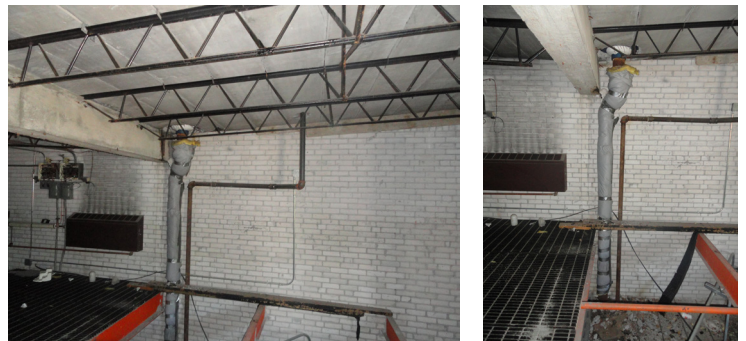
Photo 12: Storm piping with poor insulation
