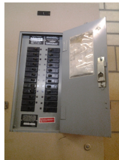
Photo 2: Examples of old panelboards in fair, operational condition
