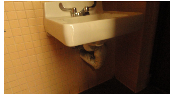
Lavatory with poor pipe insulation
