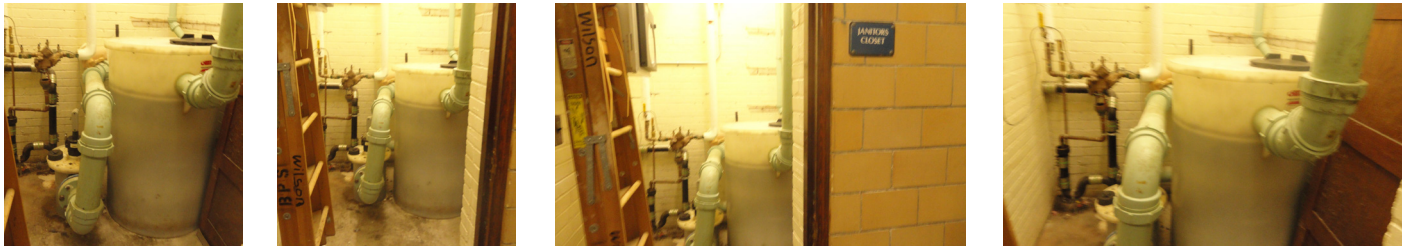
Photo 12: Acid neutralization tanks
