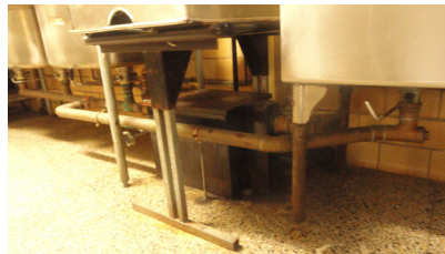
Photo 9: Waste piping installation at triple pot sink and prep sink
