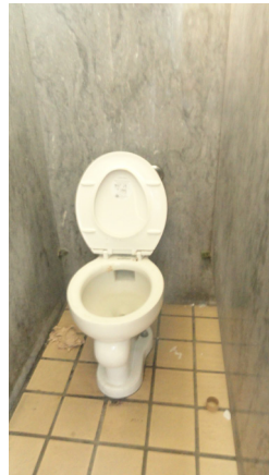
Floor mounted water closets with manual flush valves
