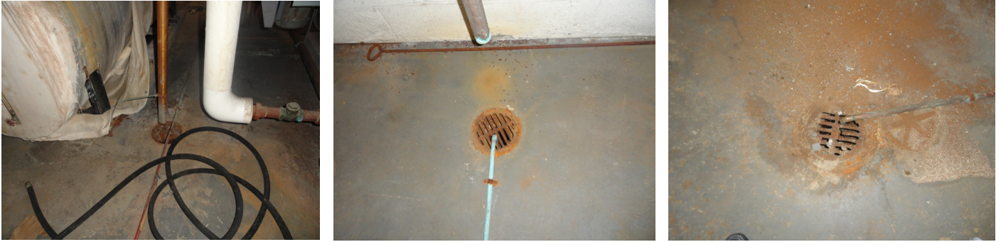
Photo 11: Rusted and deteriorating floor drain covers
