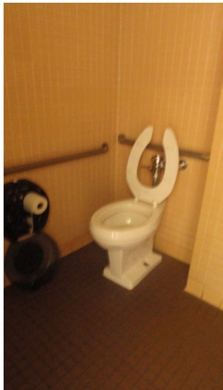
Floor mounted water closets with manual flush valves
