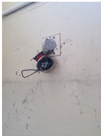
Exposed low voltage cabling
