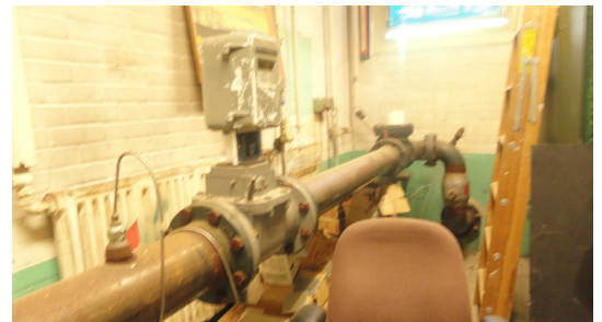
Photo 7: Gas service, gas meter and piping in the boiler room
