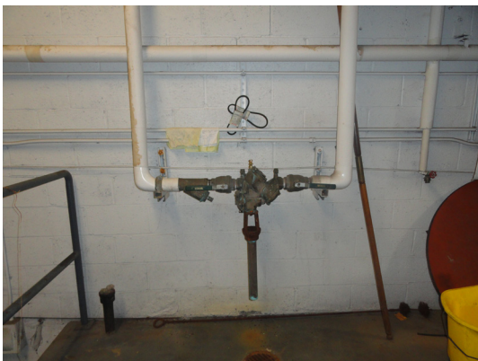
Photo 3: RPBP for HVAC make-up
