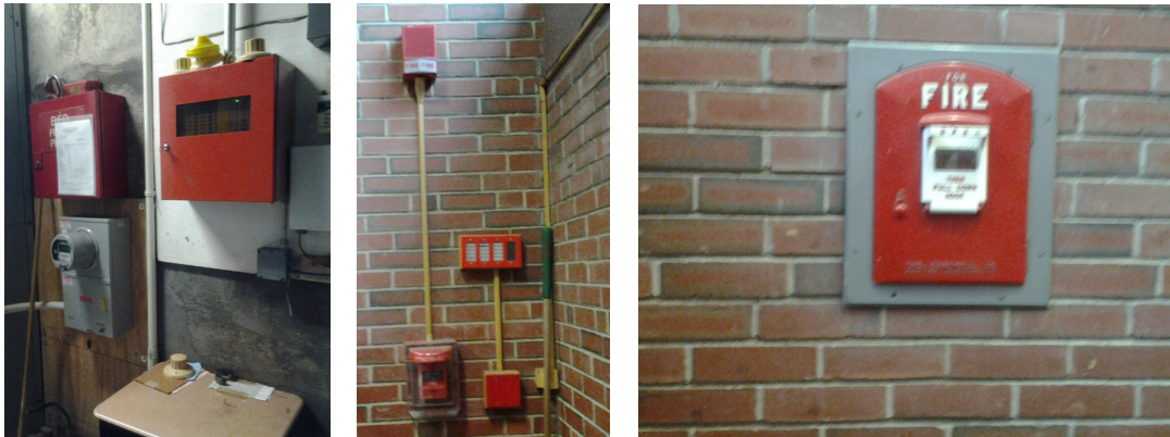
Photo 11: Existing FACP and associated equipment
