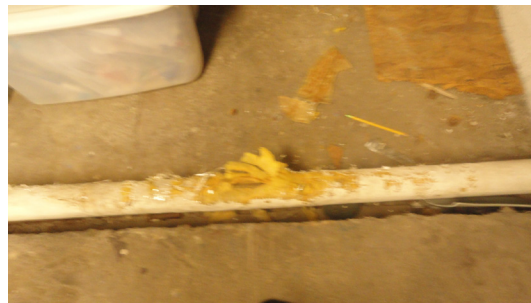
Photo 2: Uninsulated pipes and poor insulation
