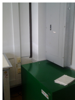
Photo 4: Example of newer panelboards and newer raceways
