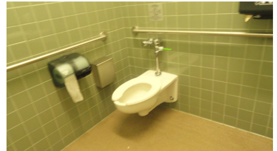
Wall mounted water closets with dual flush valves
