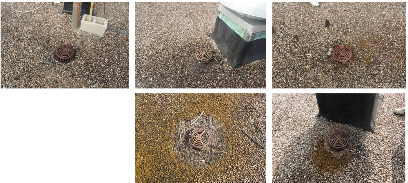
Photo 13: Roof drains and domes
