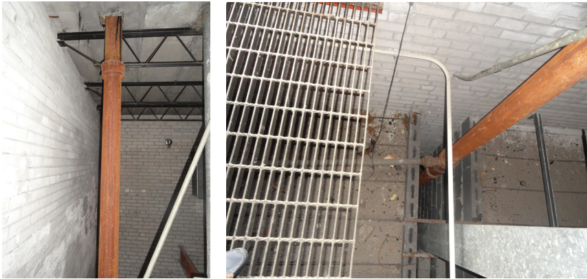
Photo 8: Rusted vent piping
