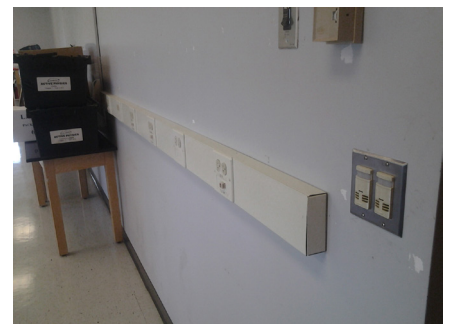
Photo 4: Example of newer panelboards and newer raceways
