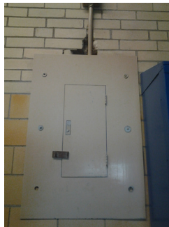
Photo 2: Examples of old panelboards in fair, operational condition
