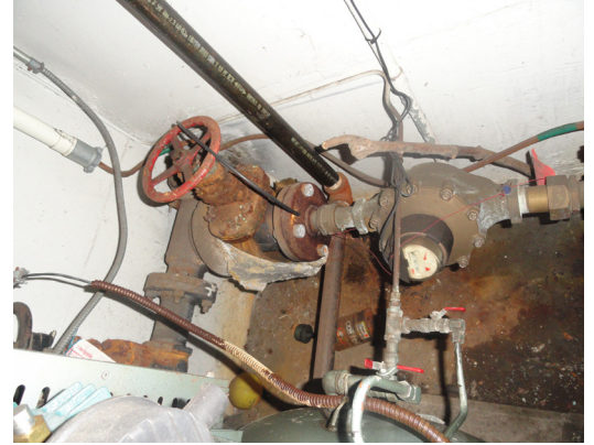
Photo 1: Domestic water service and water meter
