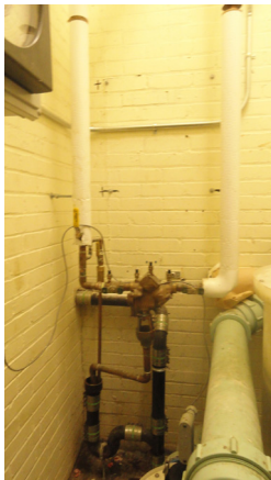
Photo 13: Backflow preventer for non-potable water system
