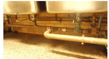
Photo 9: Waste piping installation at triple pot sink and prep sink
