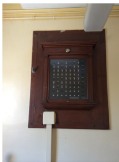
Photo 12: Original paging system wall box
