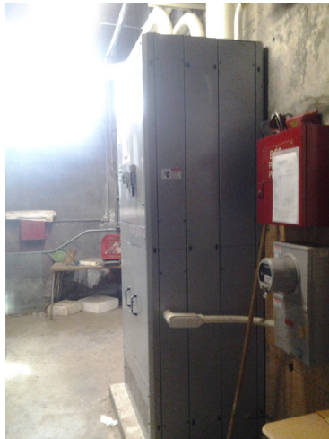
Photo 1: New main distribution equipment and utility meter
