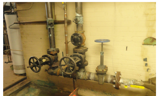
Photo 3: Leaking cold water riser
