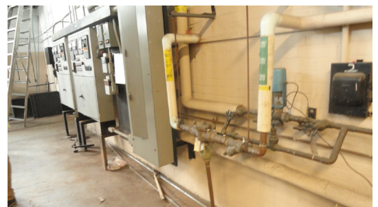
Photo 4: RPBP for HVAC make-up
