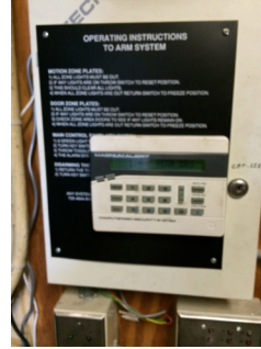
Photo 2: Intrusion detection panel
