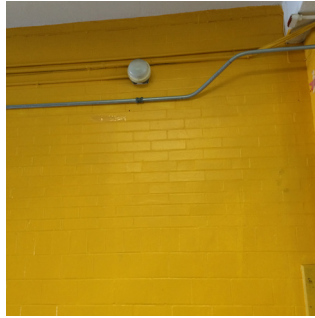
Photo 1: Wall-mounted motion sensor
