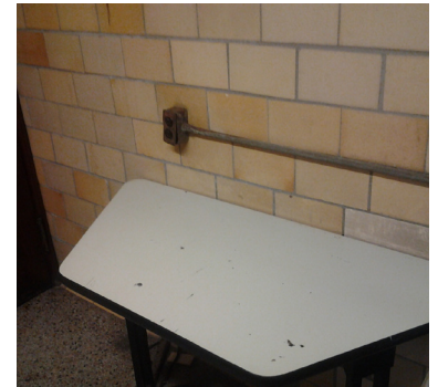
Photo 6: Example of non-GFI receptacles in the kitchen areas
