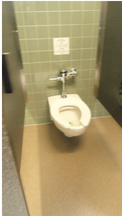
Wall-mounted water closet with manual flush valve
