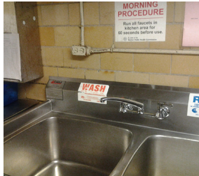
Photo 6: Example of non-GFI receptacles in the kitchen areas
