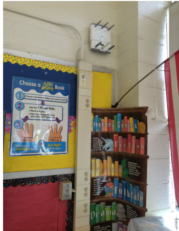
Typical classroom raceway and access point configuration
