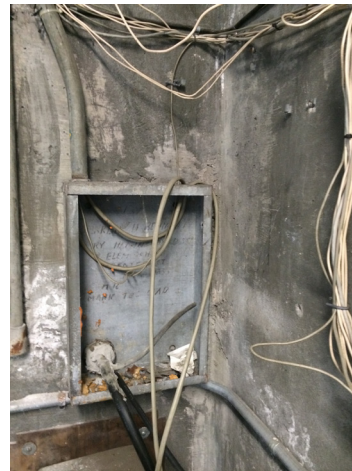
Wall-mounted communications cable pull box
