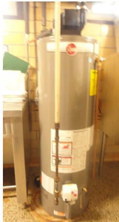
Photo 6: Gas-fired water heater in the kitchen
