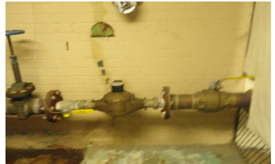
Photo 1: Domestic water service and water meter
