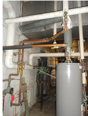
Photo 4: Gas-fired water heater in the boiler room
