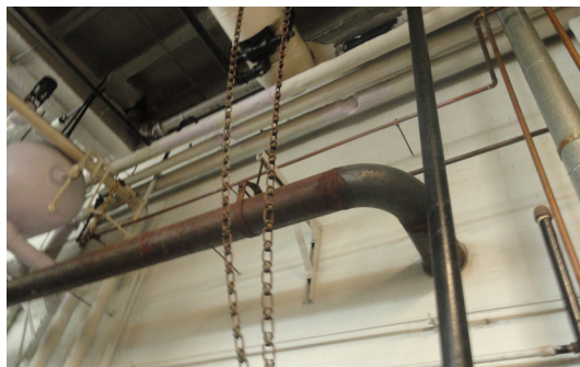
Photo 2: Uninsulated Pipes
