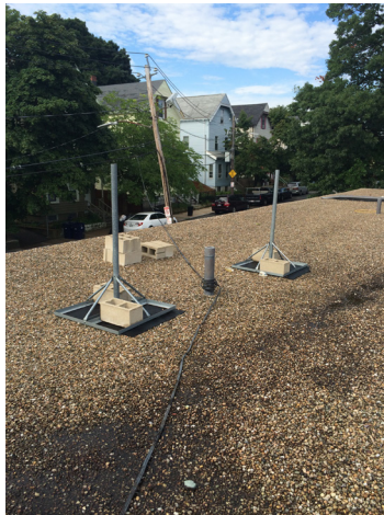
Abandoned CATV trunk cable
