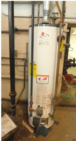
Photo 5: Gas-fired water heater in the boiler room
