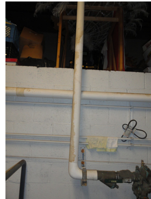
Photo 1: Domestic water service and water meter
