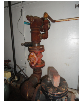
Photo 6: Gas service in poor condition
