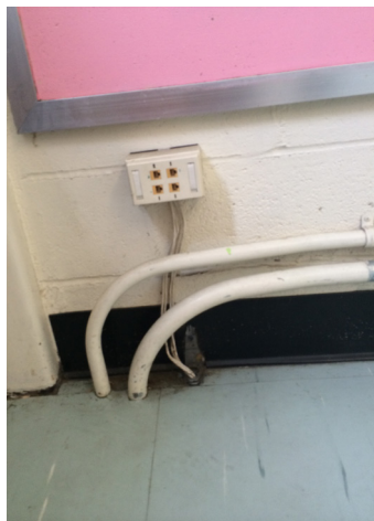
Exposed low voltage cabling
