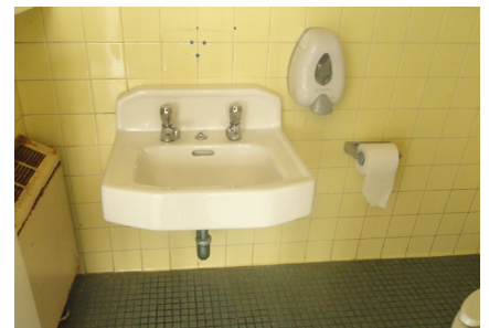
Photo 16: Non-ADA, ADA compliant lavatories and without pipe insulation
