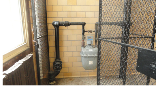
Photo 8: Gas service, gas meter and piping in the kitchen area
