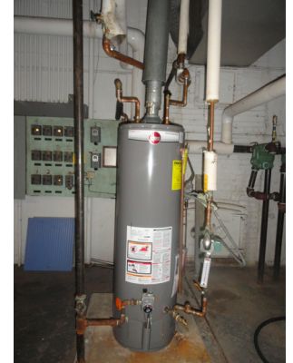
Photo 5: Uninsulated pipes and poor insulation
