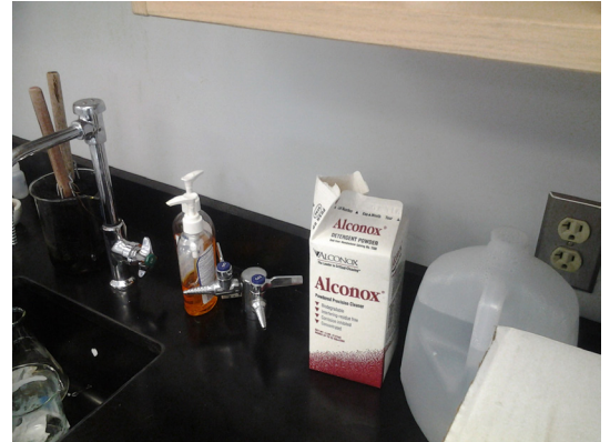
Photo 5: Example of non-GFI receptacles near sinks in science labs
