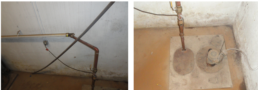
Photo 9: Existing sewage ejector
